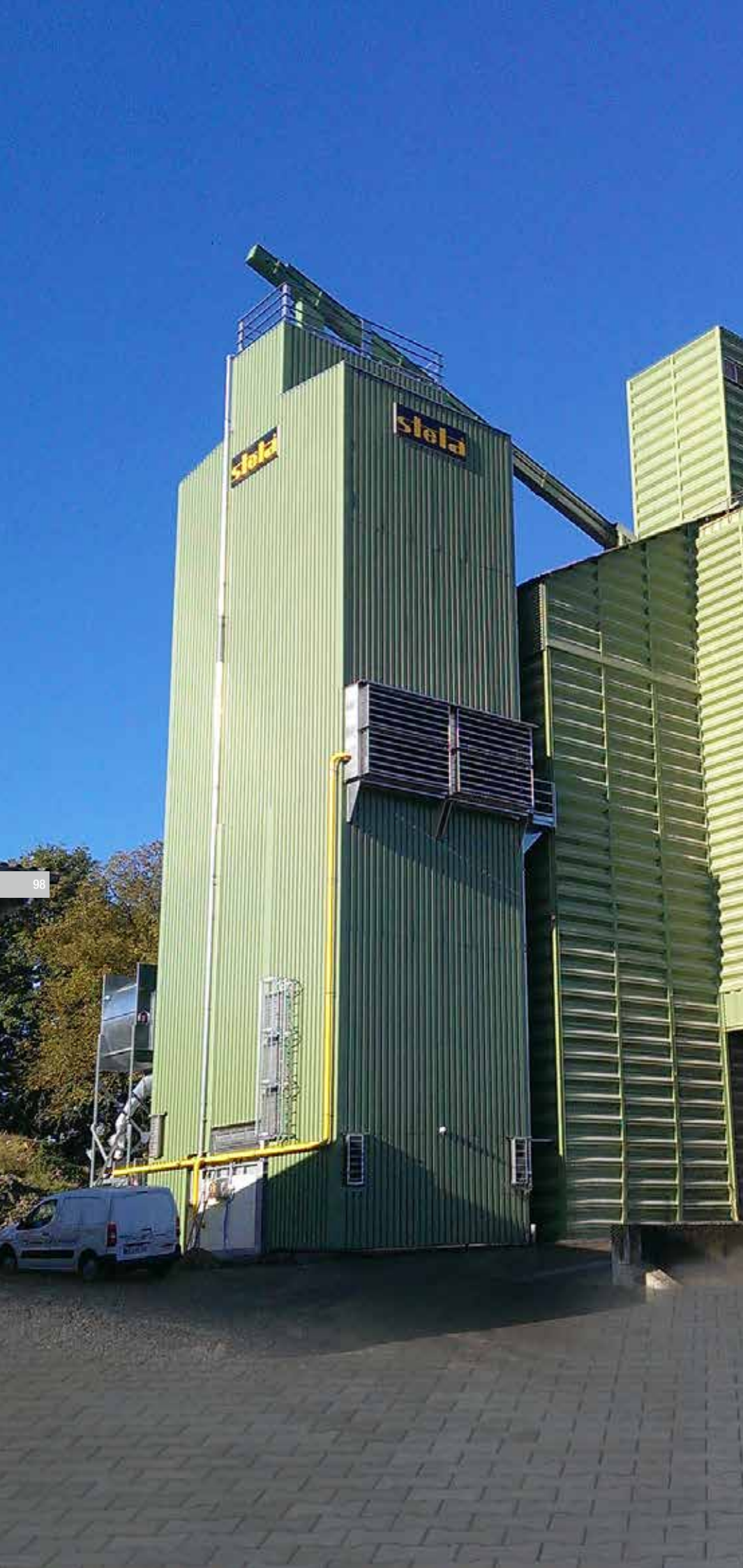
Feuerstein France, Durmenach MDB-XN 2/17-SB 2013 corn: 35.0 t/h from 35% to 15%
