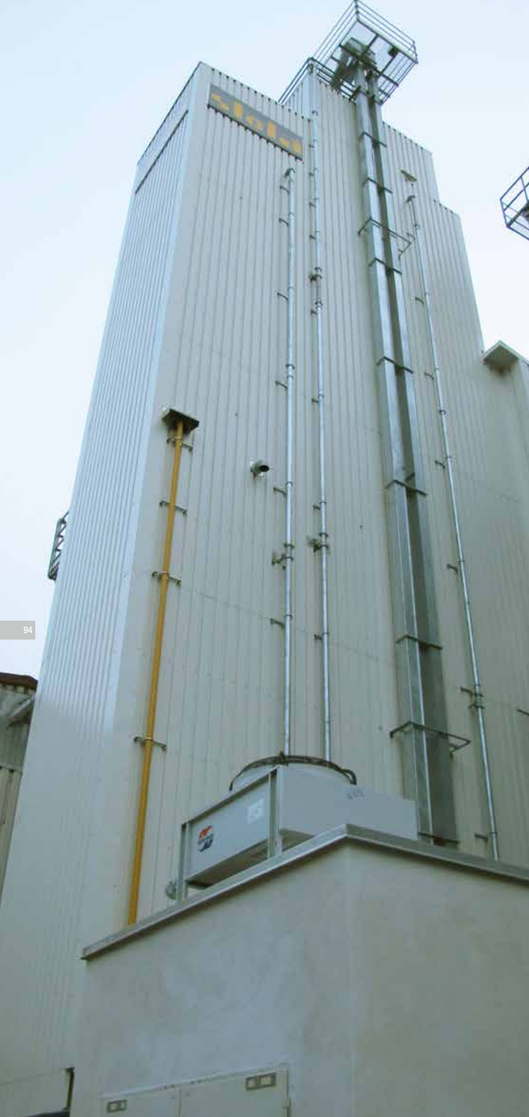
Lagerhaus Eichinger Germany, Tann MDB-TN 1/17-SB 2014 corn: 10.0 t/h from 35% to 14%
